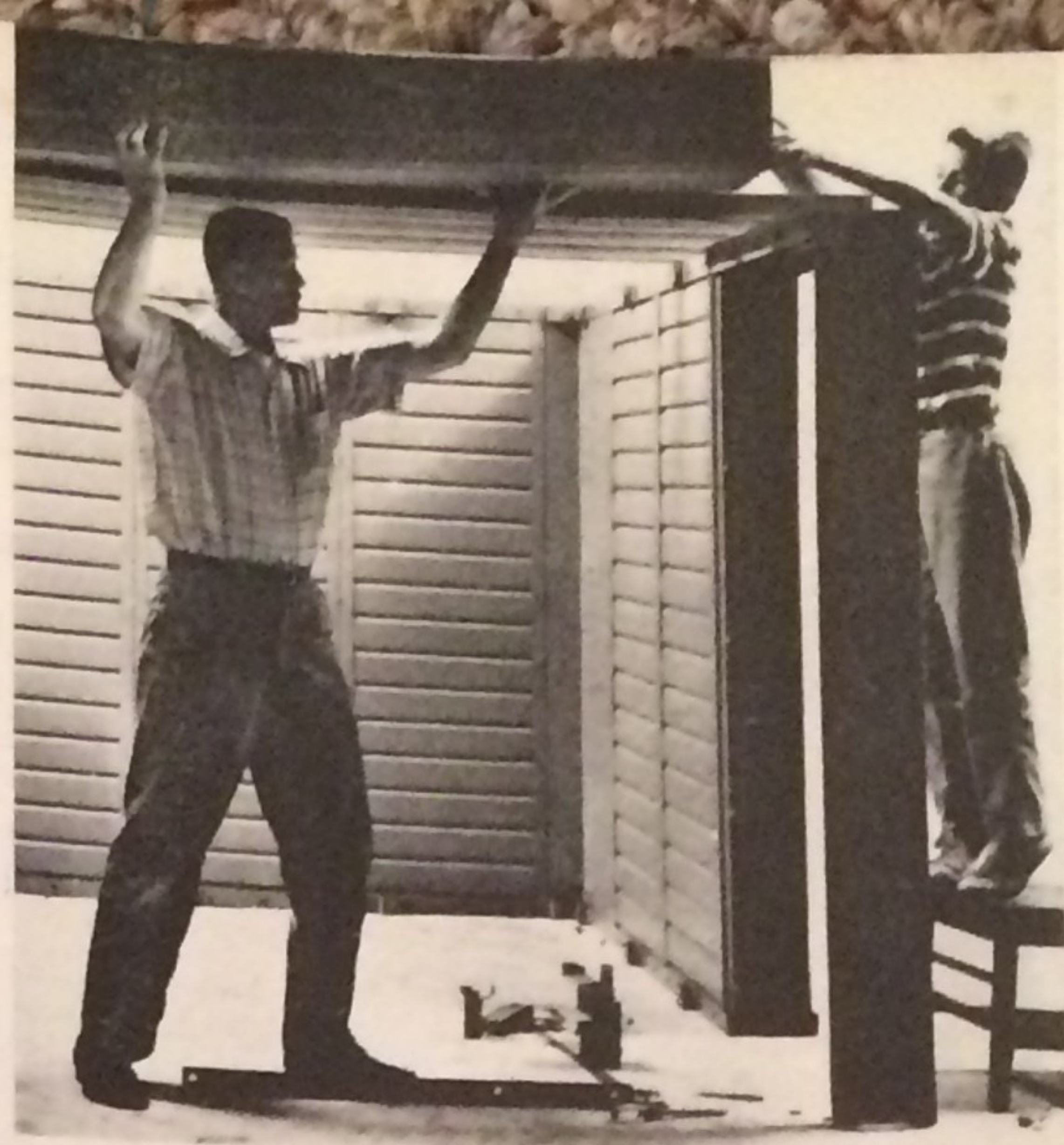
RAISING THE ROOF. With walls and door frame in position, the Carlsons place hollow section of ceiling next to crossbar. Each section of wall and roof will be filled with sand and gravel to add to strength and shielding of the shelter.
