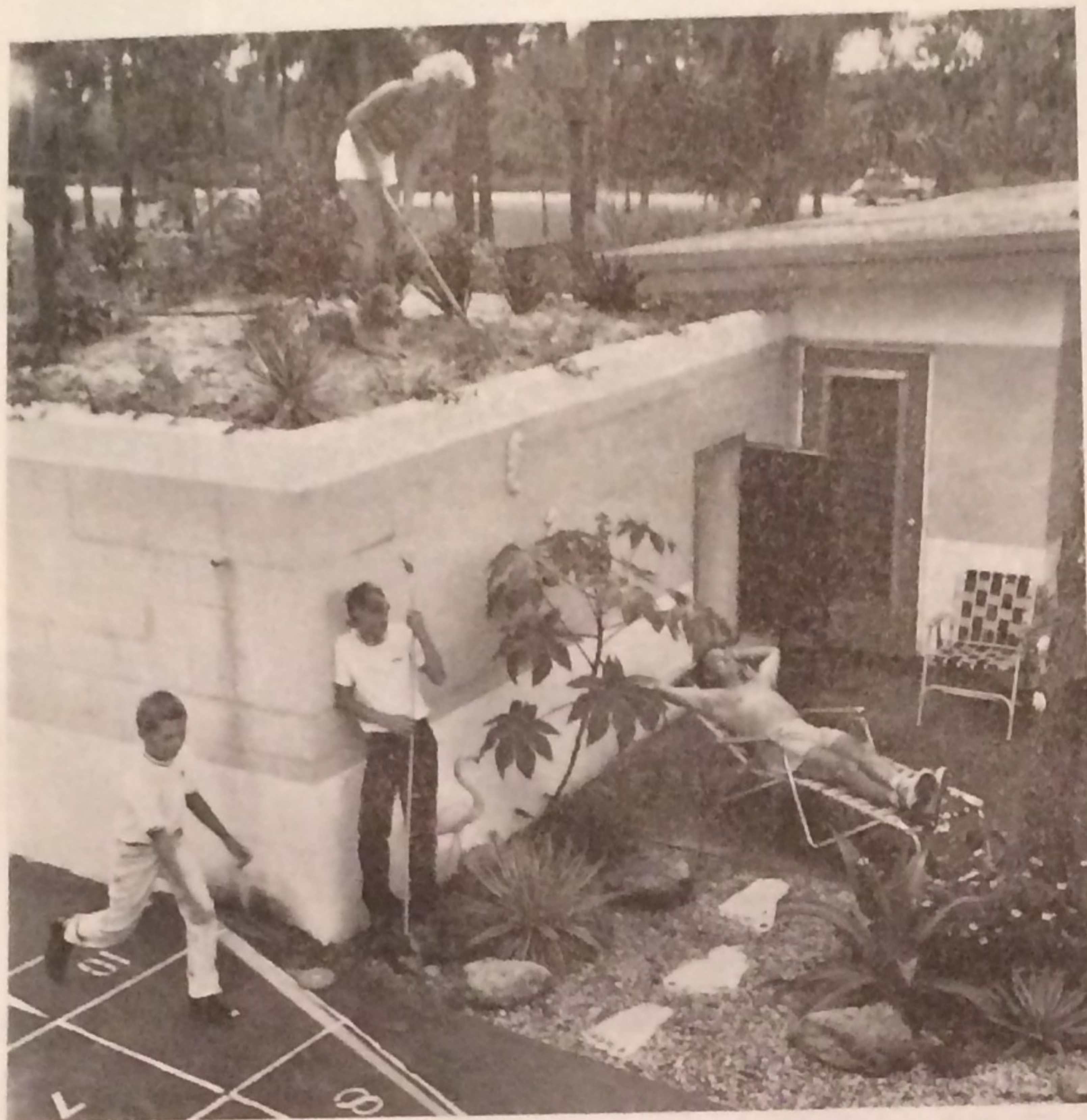
ATTRACTIVE ADDITION. In Orlando, Fla. Doug Bartholow built concrete-block shelter as annex to his house. Here family relaxes in patio as Mrs. Bartholow tends garden on roof.
