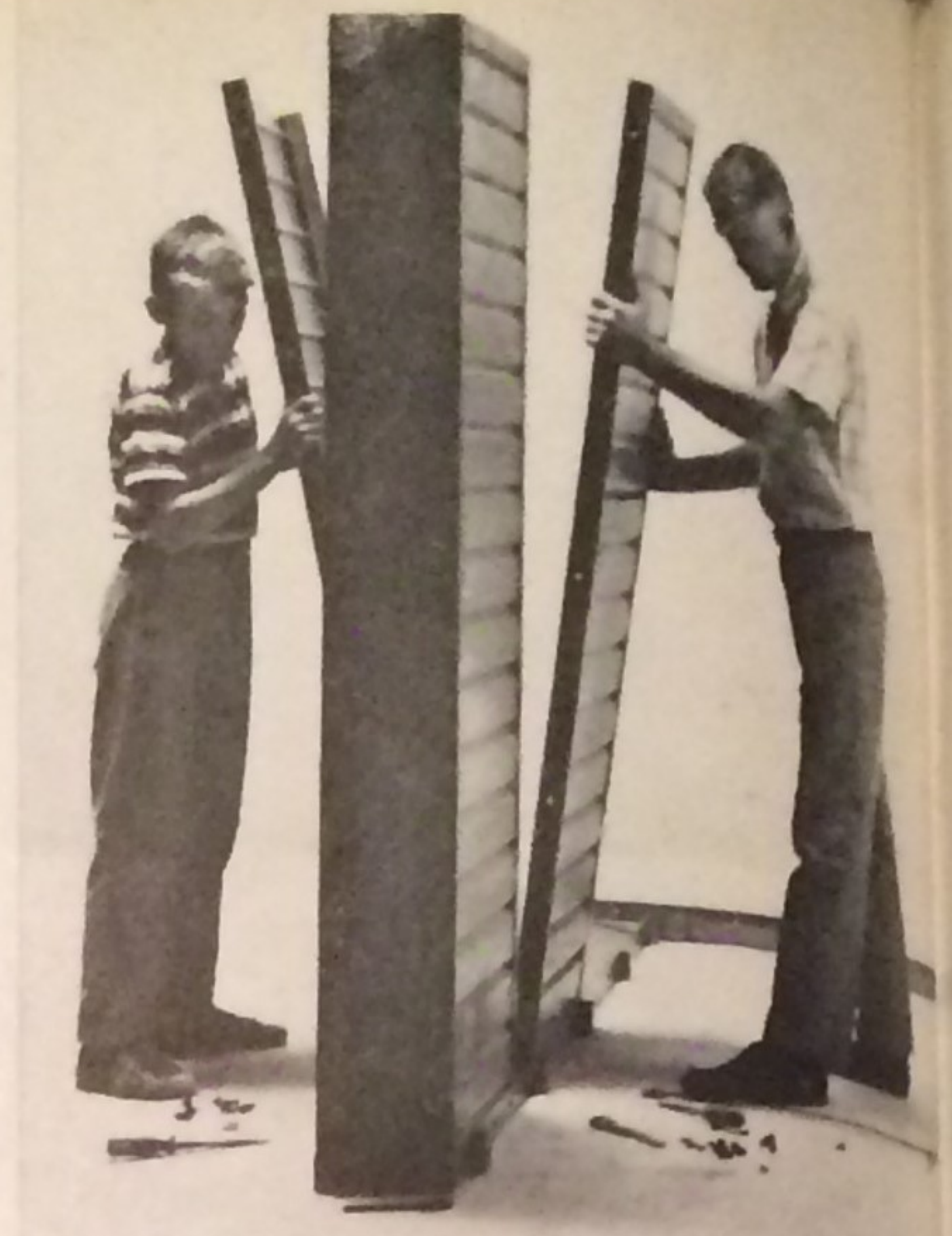
ERECTING WALL. With end piece of hollow wall in place, Carlson and his son start next segment by anchoring pieces which they will bolt together.
