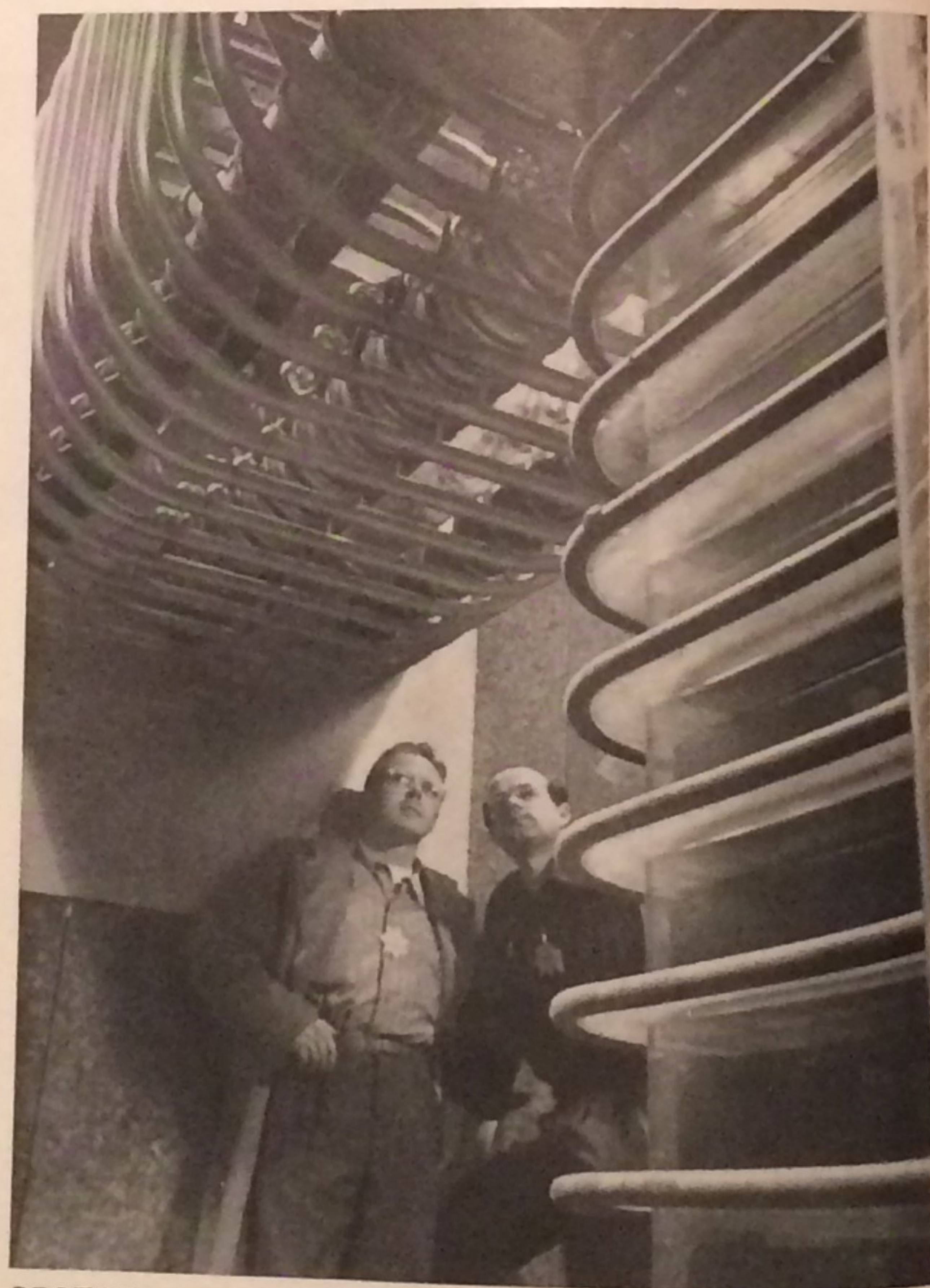
PROTONS ARE BOOSTED to 500,000 electron volts by charges generated in base of Cockroft-Walton machine. Hoops are voltage distributing rings which help pass protons down gun (above scientists) at rear of machine.
